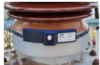
» UHF Bushing Sensor
